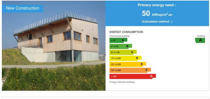
Building Type : Factories Construction Year : 2014 Delivery year : 2014 Address 1 - street : 27940 AUBEVOYE, France Climate zone : [Cfb] Marine Mild Winter, warm summer, no dry season. Net Floor Area : 710 m<sup>2</sup> Construction/refurbishment cost : 1 775 000 € Number of Installed Kw : 2 Installed Kw Cost/m2 : 2500 €/m<sup>2</sup>
