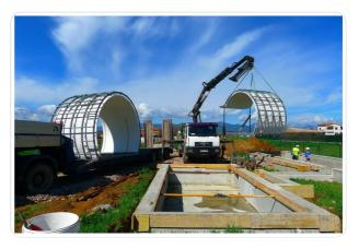
The GRC, which is the acronym in English of "Glassfibre Reinforced Cement" is a composite material, consisting of a matrix of reinforced concrete mortar with glass fibers resistant to the mortar's alkalis. The matrix is formed by a gray cement mortar CEM I 52,5 R or white BL II 42.5 R, with resistances of 52.5 and 42.5 N / mm2 respectively, and sand of silicon with a content of Quartz (SiQ2) greater than 96% of the weight of the san
