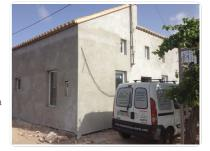
As a result of its expanded polystyrene composition the SATE system is an insulation panel that provides thermal insulation on the exterior of the home. It also has a reinforced lining and acrylic mortar.
