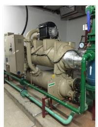
exhaust air, it can reach a higher operation efficiency, the comprehensive energy efficiency could be 20% higher than that of the conventional chiller + water pump + cooling tower system. It can run separately and bear less indoor heat load, reduce time and cost of chiller performance.
