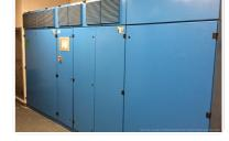
electrical current of the network, which accumulate sufficient inertia in the event of a power outage or disconnection of the network. In this way, they can continue to produce electricity without interruption for high-consumption sensitive equipment such as field lighting, media and TV cabinets, giant screens, the time that diesel emergency generators take over the network.
