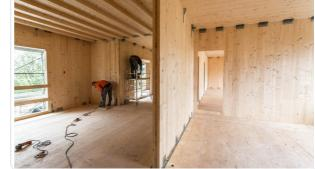
and composed of wooden elements in 5 layers cut by numerical control machines, do not contain phenolic glues and are mounted with dry plates and titanium screws.
