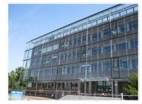
according to the terms of environmental regulatory, bioclimatic skin turns cold climate near the surrounding when it's hot and warm when it's cold. And the buffer space created between the glass skin and the existing façade allows energy performance and occupant comfort. In addition to maintaining the large openings of the buildings without reducing their surfaces, we make generous natural light in all classrooms while renewing the interior comfort without changing the medium.
