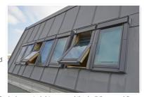
performances contribute to reducing heating needs. In summer, the automatic opening of motorized INTEGRA® windows at night can cool the building, avoiding the need for an energy-intensive air conditioning. • Life cycle: The wooden windows VELUX INTEGRA are the subject of a specific Environmental and Health Data Sheet, which can appreciate as accurately the environmental performance of the project.
