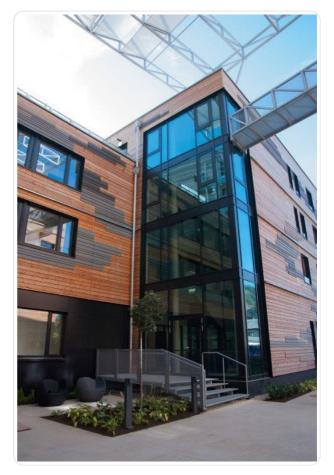
Uf value (> =) 0.7 Min. View width 50 mm Max. Glass thickness 64 mm Max. mass 700 kg statics 7160.6 cm4 surfaces powder Air permeability AE900 Water tightness
