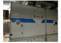
In the actual operation, the fresh air handling unit operates within the design range, the unit total air volume and power consumption per unit wind volume have been tested, and both can meet the design as well as the limit requirements, means that the equipment system performs in good condition.
