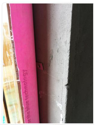
heat-breaking bridge anchor
