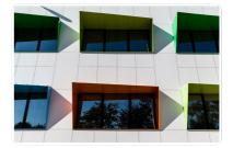
Rockpanel were used to achieve the cladding of the existing building and extension, but also to make the sunscreens that provide the colored buttons on the existing building. In addition to their environmental benefits (BRE label A + / A), Rockpanel allowed to reproduce on the facade identity colors of society, through collaboration with Akzo Nobel has provided adequate paint.
