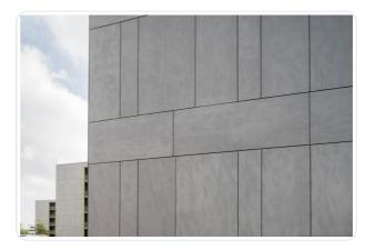
The buildings were clad in Eternit panels on the majority of their facades. This had the objective of increasing the durability of the building in time and reduce maintenance requirements. Only the facades of the protected walkways were coated weatherproof. It was a decision dictated by reasons of cost, since it is social housing.
