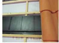
The system is placed between the tiles and the roof underlay screen in the thickness of the roof, it is connected by a tube to the heat pump of water heater. The complete system enables to lower the power consumption of the heat pump of water heater.
