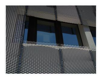
Perforated plate was used on top of the windows, reducing by 30% the incidence of the sun setting over the holes.
