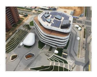
about 52 kWp, and the average annual power generation is 48623 kWh, accounting for 10-15% of the total passive electricity consumption.
