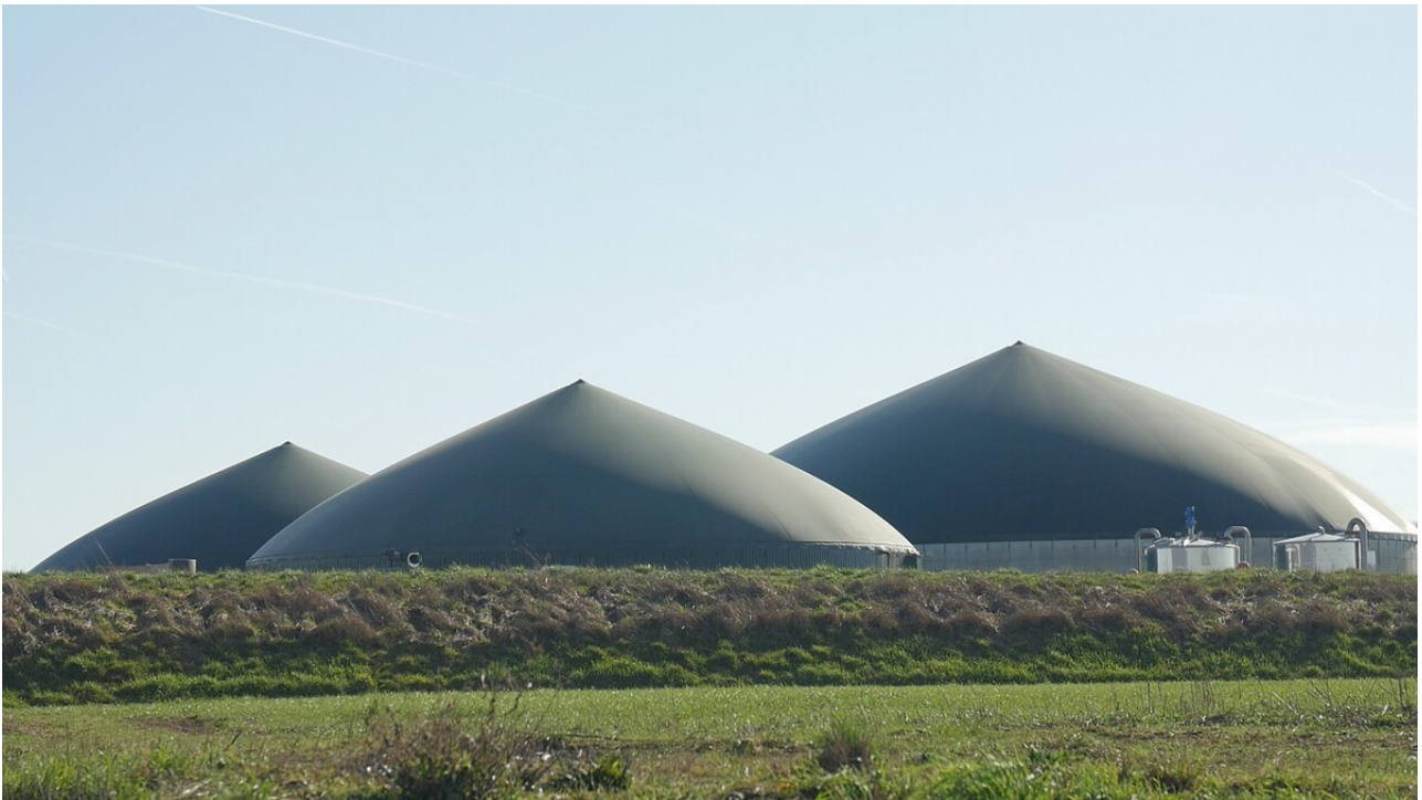
— Example of a biogas plant - photo credit: GRDF
