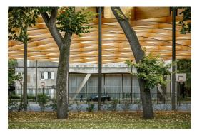
Upstream, Ivan Bloch at CBT made long calculations. This does not bother him, specialist that he is in geodesic structures. He had to anticipate the deformations and transmit the correct manufacturing data. Downstream, once the structure was laid in the summer of 2021, temporary cables compressed it and the meticulous and slow laying of the membrane gradually relieved the action of these cables. It is better to leave the installation of the membrane to specialists.
