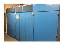
In the event of a breakdown of the traditional network, 2 dynamic inverters of 625 kVA each take up the load, useful for the continuity of the event, waiting for the start of the 3 generating sets of 800 kVA. The dynamic inverters ensure continuity for one minute, thanks to very large inertia magnetic flywheels driven by the
