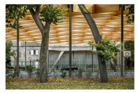
Upstream, Ivan Bloch at CBT made long calculations. This does not bother him, specialist that he is in geodesic structures. He had to anticipate the deformations and transmit the correct manufacturing data. Downstream, once the structure was laid in the summer of 2021, temporary cables compressed it and the meticulous and slow laying of the membrane gradually relieved the action of these cables. It is better to leave the installation of the membrane to specialists.
