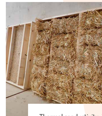
Wall insulation by 100 to 150 mm rectangular bales
