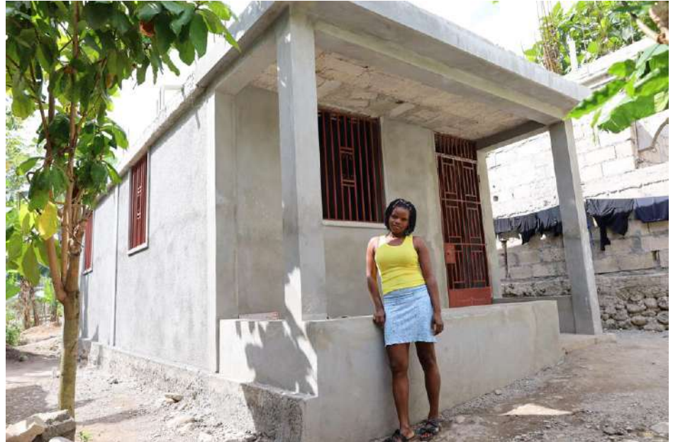
Naomie Goubert in front of her retrofitted home in Chantal, Haiti
