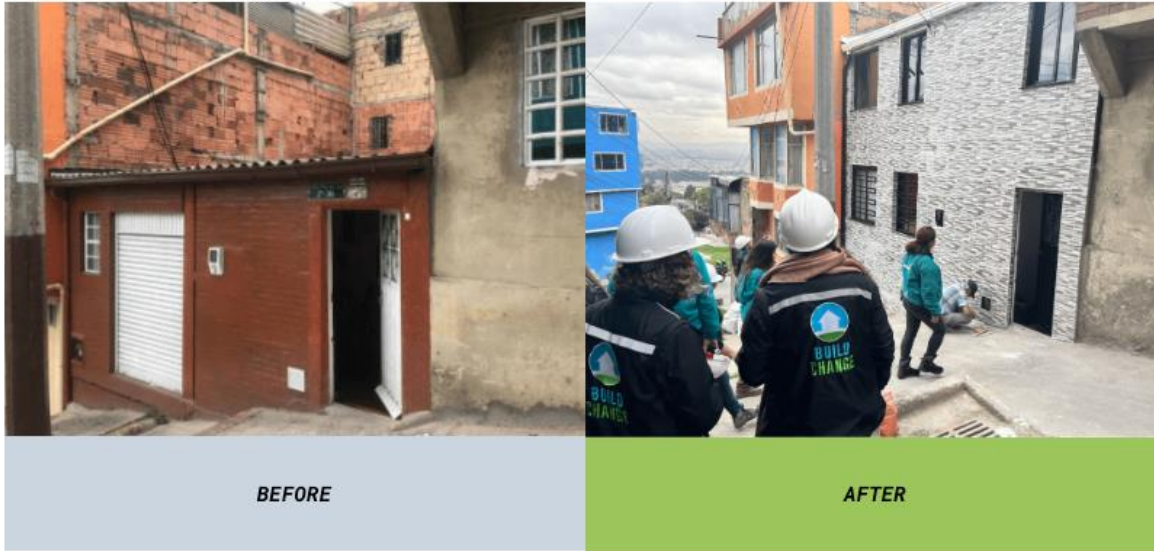
Ercilia Suarez's house before and after retrofit and vertical expansion under the city of Bogotá's Plan Terrazas program, supported by technical assistance from Build Change.
