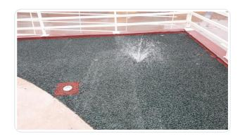
of a draining floor covering. At SCL, we connected the Hydromedia tiling to a retention tank for storage and recycling of rainwater and wash water from the showroom.
