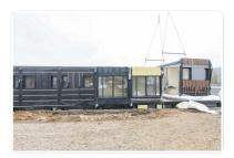
After years of research and development, Smart Module Concept has developed its own modular construction system. Our buildings are 95% factory built in order to guarantee quality, delivery time and budget. Constructed of modules that can be combined in different ways, our constructions meet the needs of space and functionality while favoring architectural quality.
