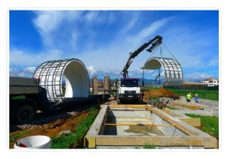
The GRC, which is the acronym in English of "Glassfibre Reinforced Cement" is a composite material, consisting of a matrix of reinforced concrete mortar with glass fibers resistant to the mortar's alkalis. The matrix is formed by a gray cement mortar CEM I 52,5 R or white BL II 42.5 R, with resistances of 52.5 and 42.5 N / mm2 respectively, and sand
