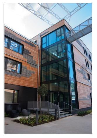
Uf value (> =) 0.7 Min. View width 50 mm Max. Glass thickness 64 mm Max. mass 700 kg statics 7160.6 cm4 surfaces powder
