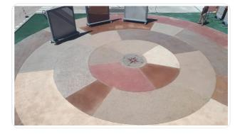
Decorative concrete, used as paving. Reinforced concrete, it plays both a structural role and a role of flooring. It exists in different finishes: polished, rock (bush-hammered), relief (deactivated), color, imprint, sand.
