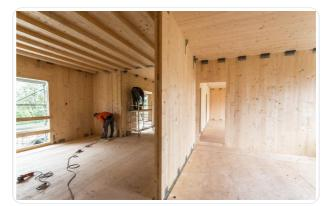
The system with load-bearing panels x-lam and composed of wooden elements in 5 layers cut by numerical control machines, do not contain phenolic glues and are mounted with dry plates and titanium screws.
