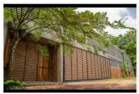
crete block screen wall provides both security and shade to the major habitable spaces. The perforated wall allows the free movement air to the internal spaces
