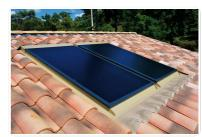
Very well accepted by the roofing company, Terreal's integration kit was developed with traditional hedging techniques and a companion of duty.
