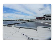
has been set up to monitor production in real time and check the efficiency of the inverters. Cleaning of the panels is carried out once a year to ensure better productivity.
