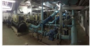
which is used for air conditioning. It does not need other heat sources to assist water heating. The comprehensive energy efficiency ratio of cooling and heating can reach more than 8.3. Compared with other conventional water-water heat pump units, such comprehensive energy efficiency ratio is about 60% higher.
