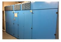
electrical current of the network, which accumulate sufficient inertia in the event of a power outage or disconnection of the network. In this way, they can continue to produce electricity without interruption for high-consumption sensitive equipment such as field lighting, media and TV cabinets, giant screens, the time that diesel emergency generators take over the network.
