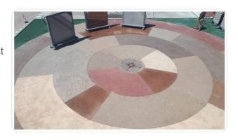
Decorative concrete, used as paving. Reinforced concrete, it plays both a structural role and a role of flooring. It exists in different finishes: polished, rock (bush-hammered), relief (deactivated), color, imprint, sand.
