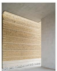
The production of rammed earth is simple, but requires an attraction to the material and know-how in formwork and compaction technology. Rammed clay is very solid, its density is comparable to concrete. Rammed earth thus works excellently as a storage mass and regulates the room air humidity in a natural way.
