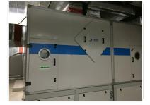
dehumidification. In winter, lake water source is used as a heat source, by use of the screw heat pump unit to provide hot water to front coil, so as to heat the fresh air.
