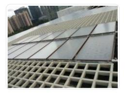
technology, with good forming quality, low thermal resistance and a service life of more than 30 years; The core is provided with the most advanced blue titanium coating in China, with high absorptivity and low emissivity; 1.2Mpa pressure test shall be conducted after the core is manufactured to ensure reliable quality of the heat collector; The frame of the heat collector is made of aluminum-magnesium alloy processed by special technology, which is elegant in
