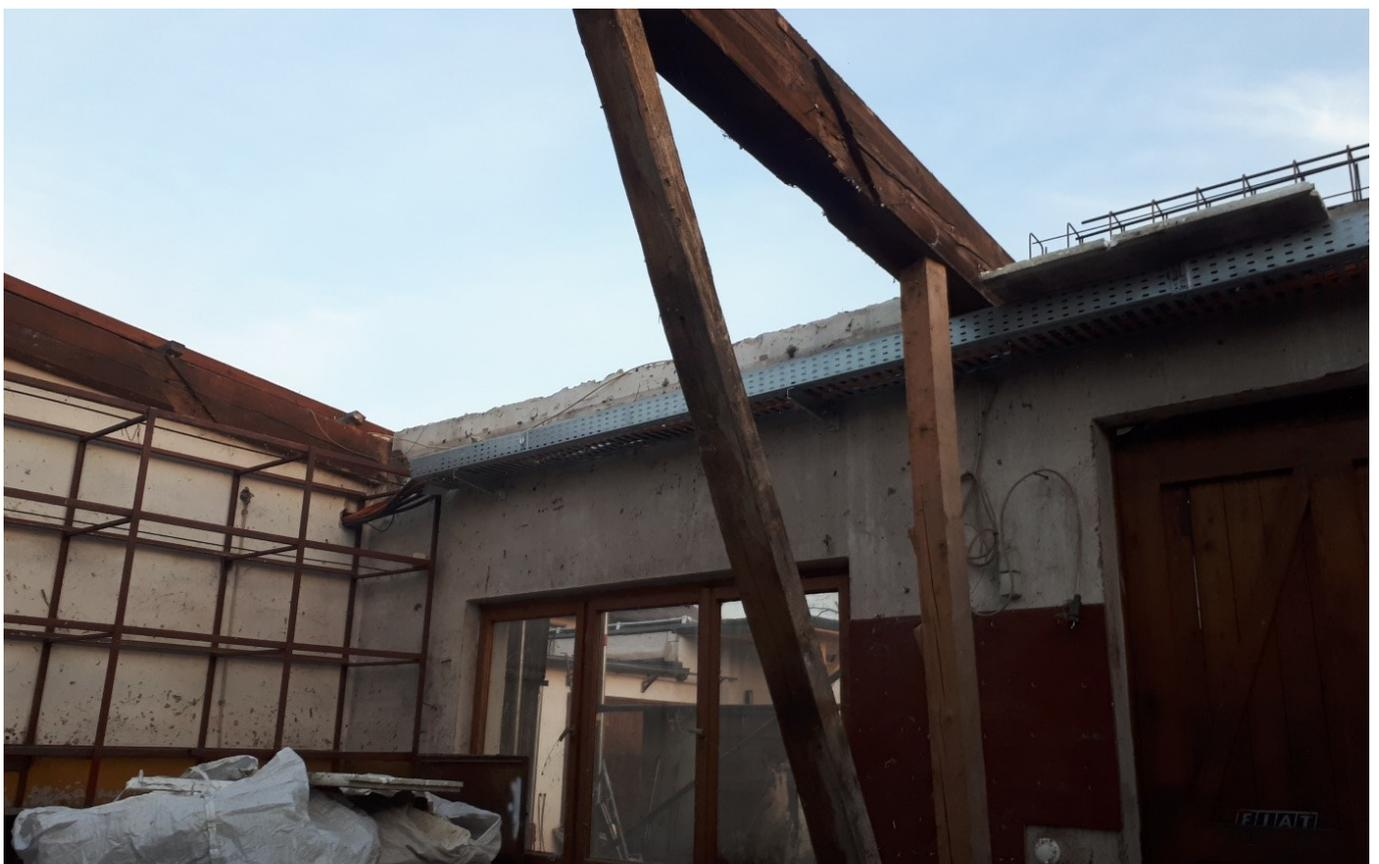
Figure 7 Safety measures for the roof structure before final and safe removal
