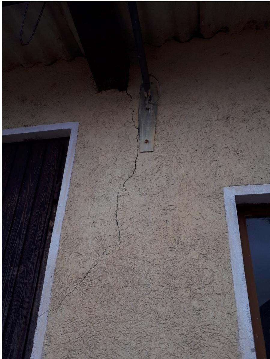
Figure 3 : Cracks in the wall due to the heavy load from the wooden beams
