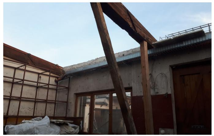
Figure 7 Safety measures for the roof structure before final and safe removement
