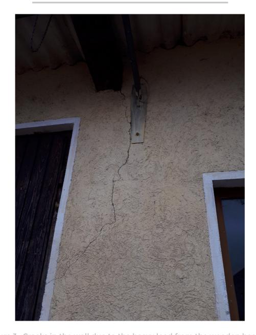
Figure 3 : Cracks in the wall due to the heavy load from the wooden beams
