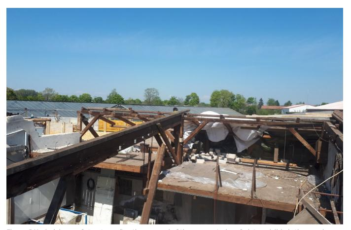
Figure 6 Underlying roof structure after the removal of the corrugated roof plates, visible is the crawl space which will later serve as the technic room for the rooftop greenhouse
