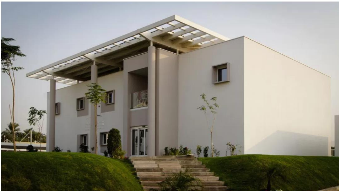
The Mohammed Bin Rashid Space Center (MBRSC) in Dubai, also a Passive House, together with the Bonn Student Residence 42! was nominated for the Green Solutions Award 2017. © MBRSC / Dubai
