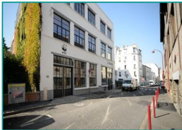
Rehabilitation of a building for WWF France headquarters, Pré Saint-Gervais, by Rabot Dutilleul Construction
