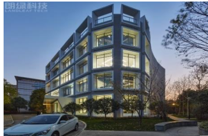
Shanghai Landsea Green Center, China – Renovation Grand Prize ©Shanghai Landleaf Construction Technology Co., Ltd.
