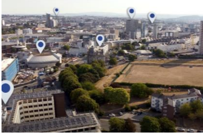
The 5 th generation heating and cooling grid of Plymouth, UK – Green Solutions Awards Grand Prize + Sustainable Infrastructure Grand Prize ©Plymouth City Council
