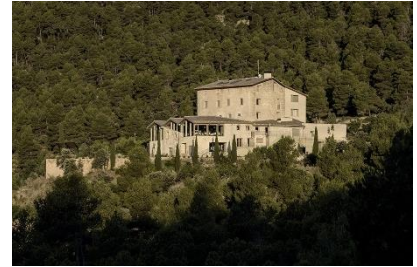
Hotel 'Mas Torre del Marqués' , Circular Economy Prize + Building User's Choice (Spain) – @Xavier d'Arquer
