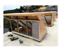
The interventions are developed through several micro actions and focus on energy rehabilitation and the improvement of housing habitability: thermal insulation on the roof, increased passive solar uptake, watertightness in carpentry, or extraction systems and control of the foul air.
