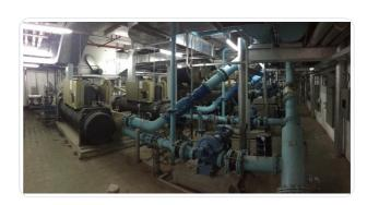
return water temperature of chilled water is 7/15°C (37.5% less energy consumption than the conventional 5°C chilled water temperature difference). The EER is 6.79, much higher than national energy efficiency level 1 (6.1). In addition, the water resistance of evaporator and condenser of the selected chiller is low. Compared with the conventional chiller, the water resistance is reduced by 40-60 kPa, which can greatly reduce the pump head and the energy consumption of water pumps.
