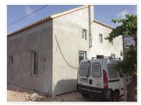
As a result of its expanded polystyrene composition the SATE system is an insulation panel that provides thermal insulation on the exterior of the home. It also has a reinforced lining and acrylic mortar.
