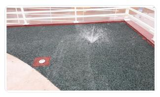
of a draining floor covering. At SCL, we connected the Hydromedia tiling to a retention tank for storage and recycling of rainwater and wash water from the showroom.
