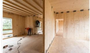
and composed of wooden elements in 5 layers cut by numerical control machines, do not contain phenolic glues and are mounted with dry plates and titanium screws.
