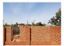
Unstabilised and made only with bio and geo-sourced materials (site soil, termite mound soil, laterite, sand, plant fibres or other), adobes are recyclable for life.
